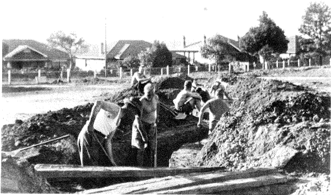
Grandfathers from the Roseville community dug trenches on the grassed area of the boys' playground. Addison Avenue is in the background, 1940.
